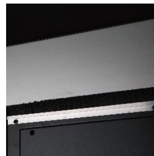
Brush all around to prevent the energy leakage.
